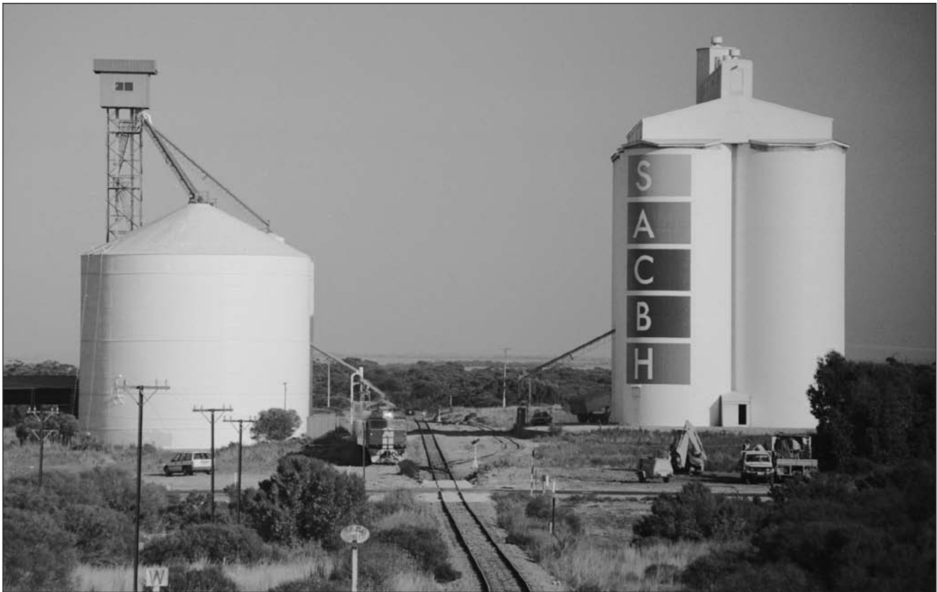
Above: NJ5 and another NJ shunt the 'new' silo siding at Kyancutta in the 1980s. The concrete silos (built 1965, extended 1969) and steel bins (built 1970) at this location are typical of those found at many Eyre Peninsula sidings.. Photo: Greg O'Brien.
