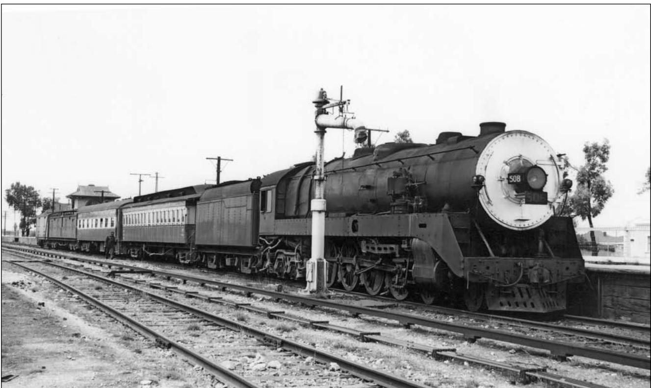
Below: 508 on train No.444 ex Pinnaroo at Taillem Bend. 508 features an extended smokebox and a pressed steel cowcatcher. The trailing vehicle, an RB type refrigerator car was normally detached at Murray Bridge; vehicles were not permitted to be trailed outside the brakevan through the Adelaide Hills section. Photo: Peter Bartrop.
