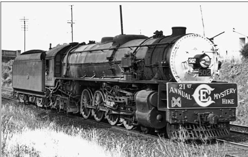
Left: 502 at Clapham in 1953 on a charter trip. The only concession to streamlining on 502 and 506 appears to be the cover over the sanding valves. Photo: National Railway Museum collection BU12682.
