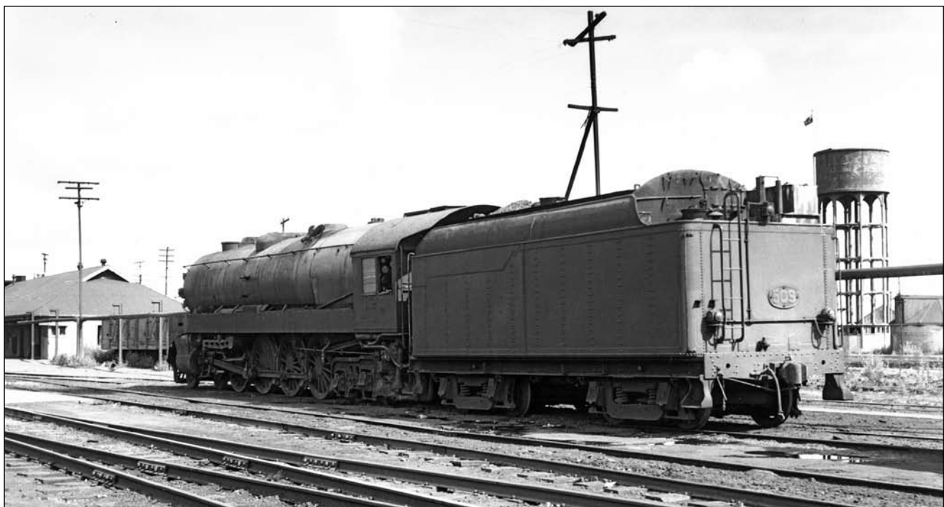
Below: Number 509 gives a good view of the rear of its tender in this shot taken at Mile End in April 1954. The reversing lamp is high above the rear deck but there is no plate showing its original position as there is on 503. The water treatment plant shows up well on this photo. Photo: A.R.Jaggard, Noel Bruce collection, National Railway Museum collection AB14757.
